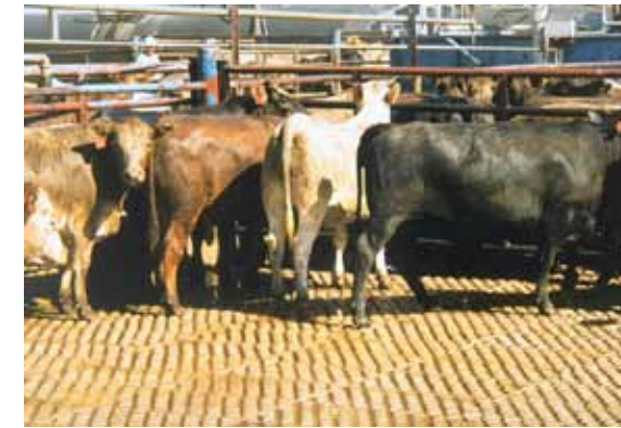
A good sample of non-slip flooring.
